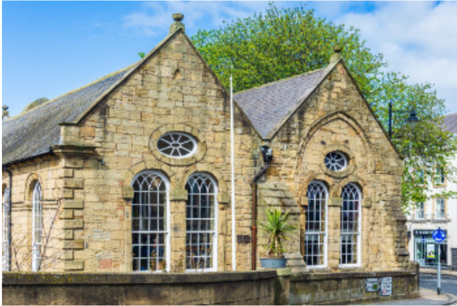
The east end of the Chantry next to the Telford Bridge: the 1738 south extension is to the left, while the original east end of the chapel (chancel) is to the right. Note how the windows on the right-hand side are set within a much larger gothic (pointed) arch. The current windows are Georgian in character to match the south extension. The gothic arch itself could be a modification as the chancel would likely have had lancet windows such as the blocked lancet around the corner on the north side of the building
