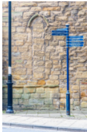
Blocked up lancet window and doorway on the north (Bridge Street) side of the Chantry
