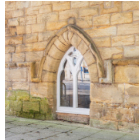
Window at street level on the Bridge Street side of the Chantry – much of the original depth of this opening will be hidden beneath street level. The window is modern having been added in 2009. Originally, this would have been the north doorway
